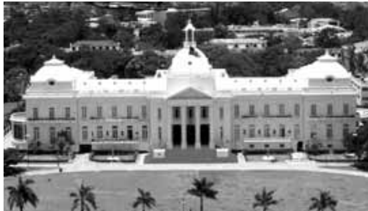
The presidential palace in Port-au-Prince collapsed after the Jan. 12, 2010.
